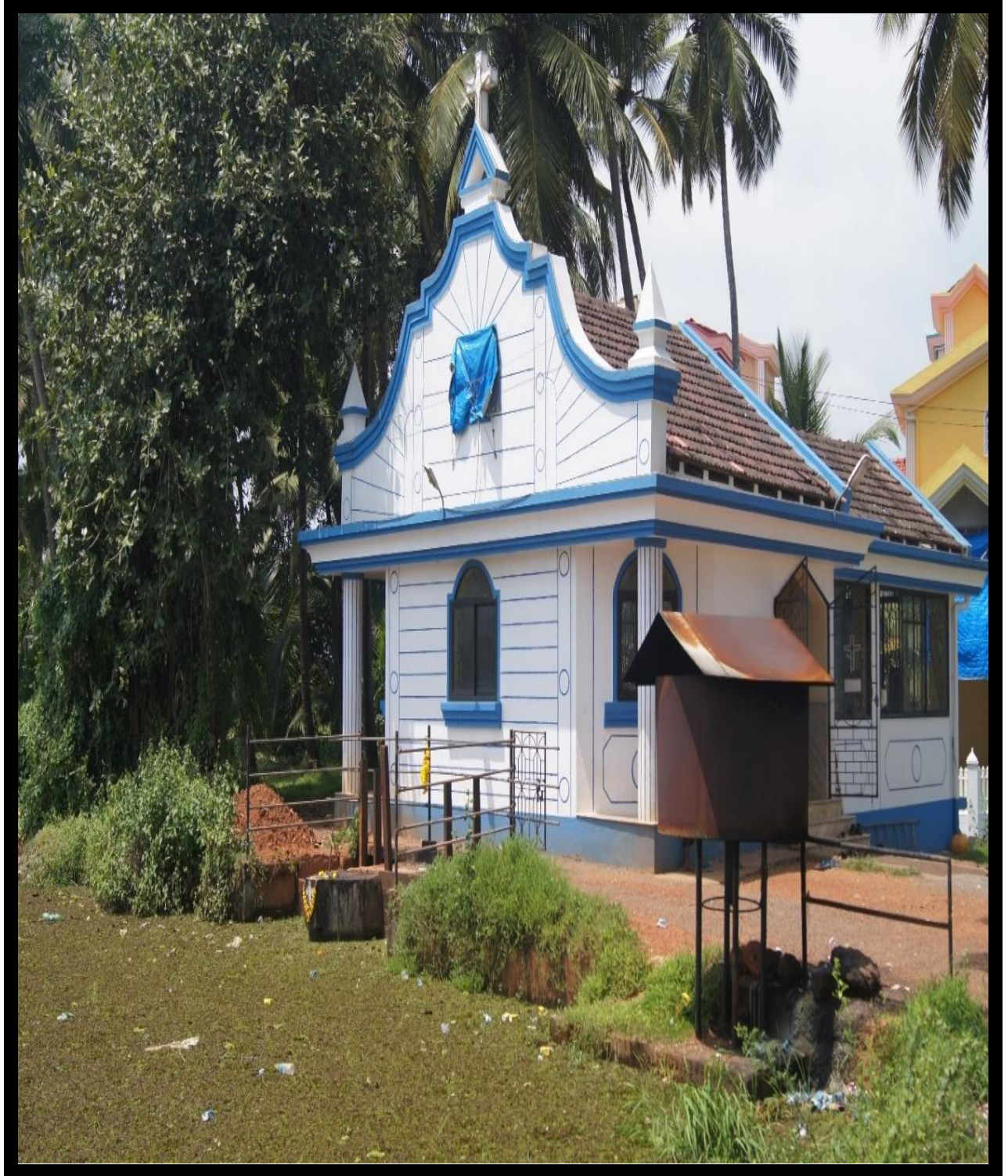
HANDI CROSS AT MAINA AND SLUICE-GATE
